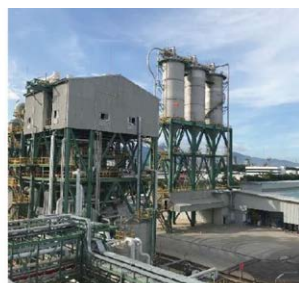
Newly built PVC manufacturing
